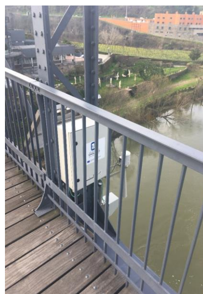
Figure 3- Carrapatelo lock limnimeter
